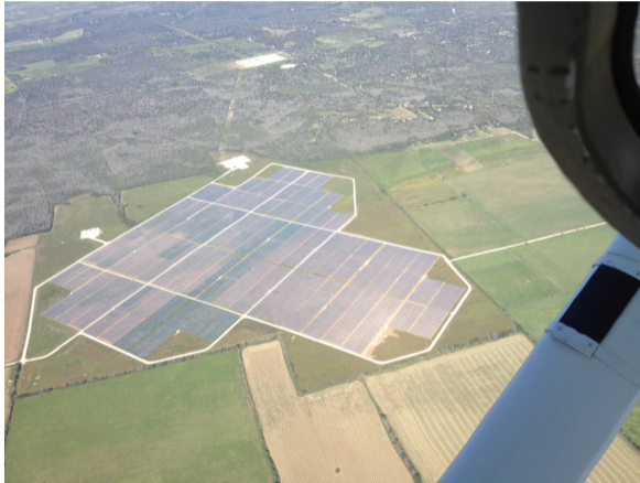
Webberville Solar Farm, Austin TX (35 MW)
